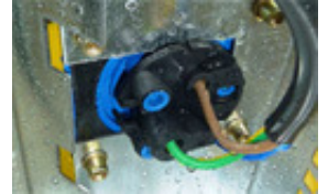
Figure 1 - rear of 230V ac connector installed to affected units
