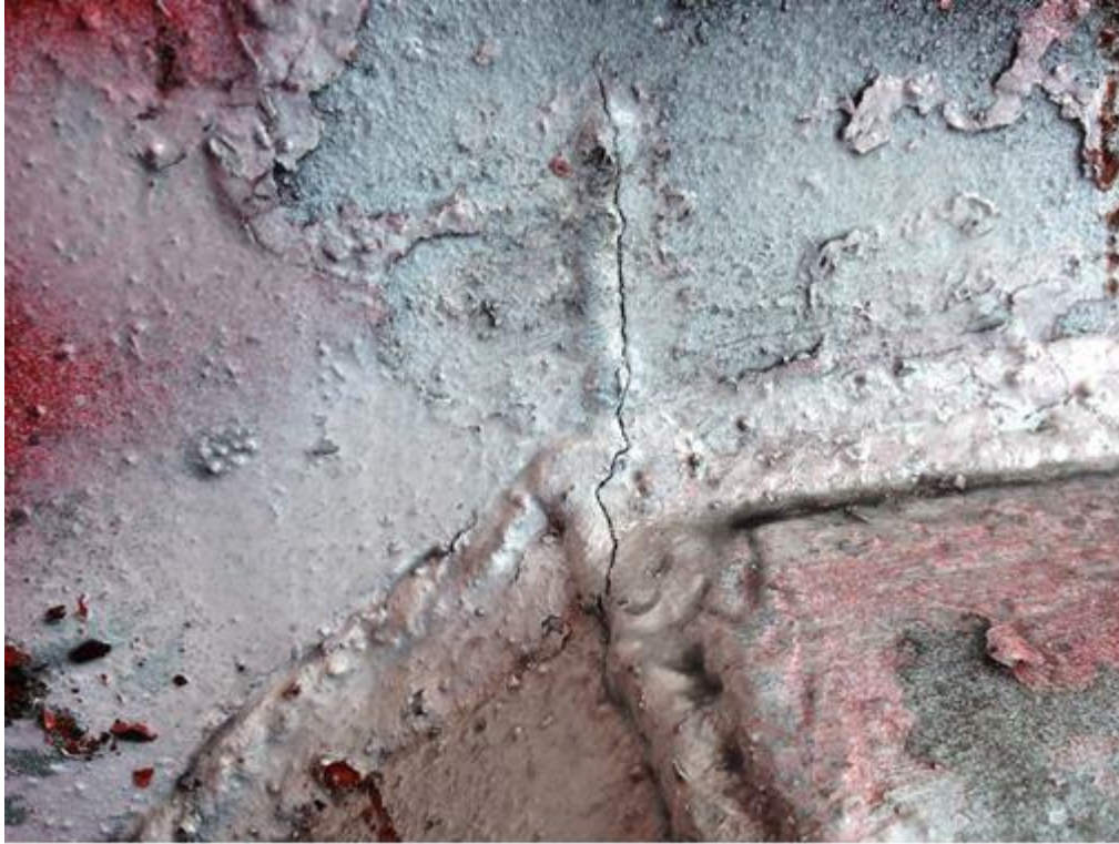
Photo 2 - 55mm crack
