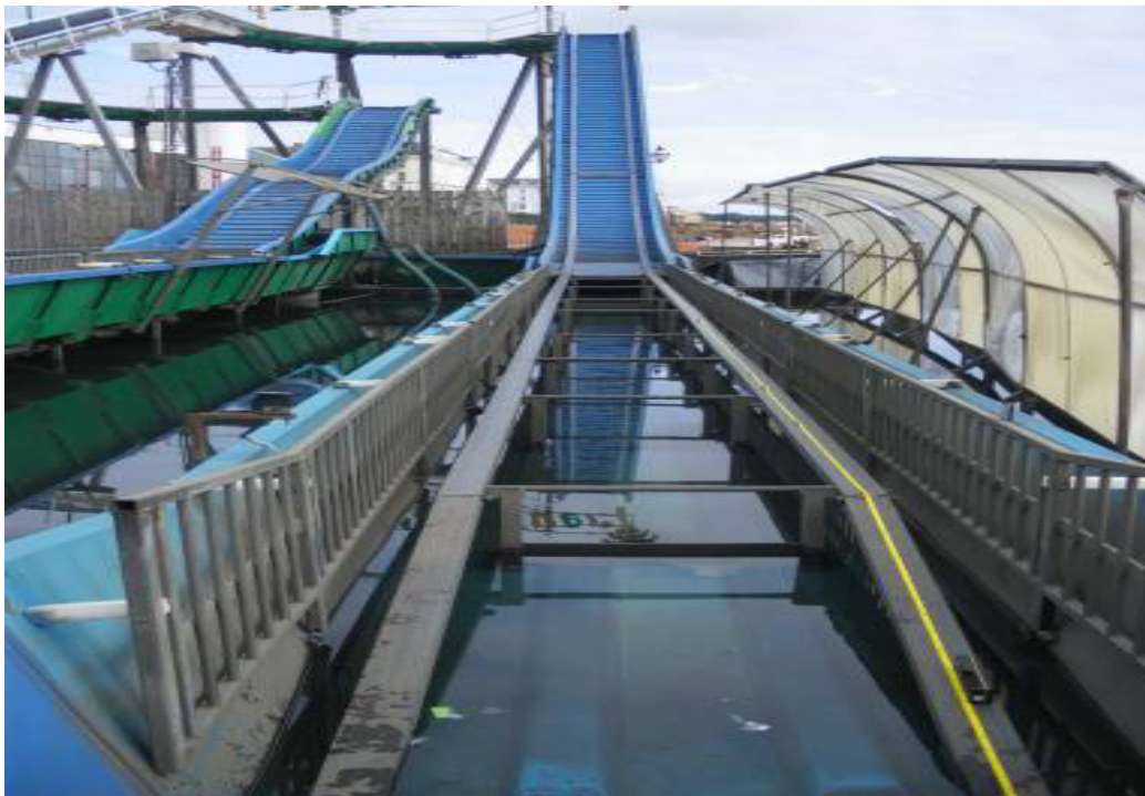
Splash tank and rails
