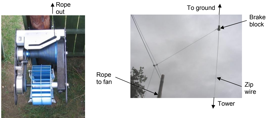
Photograph showing the rope as it is pulled out of the fan brake and connection from the brake block on the zip wire to the fan (from below).
