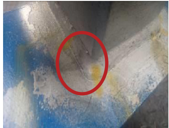
▲ Reverchon Crazy Mouse support column track allocation cone cracking
