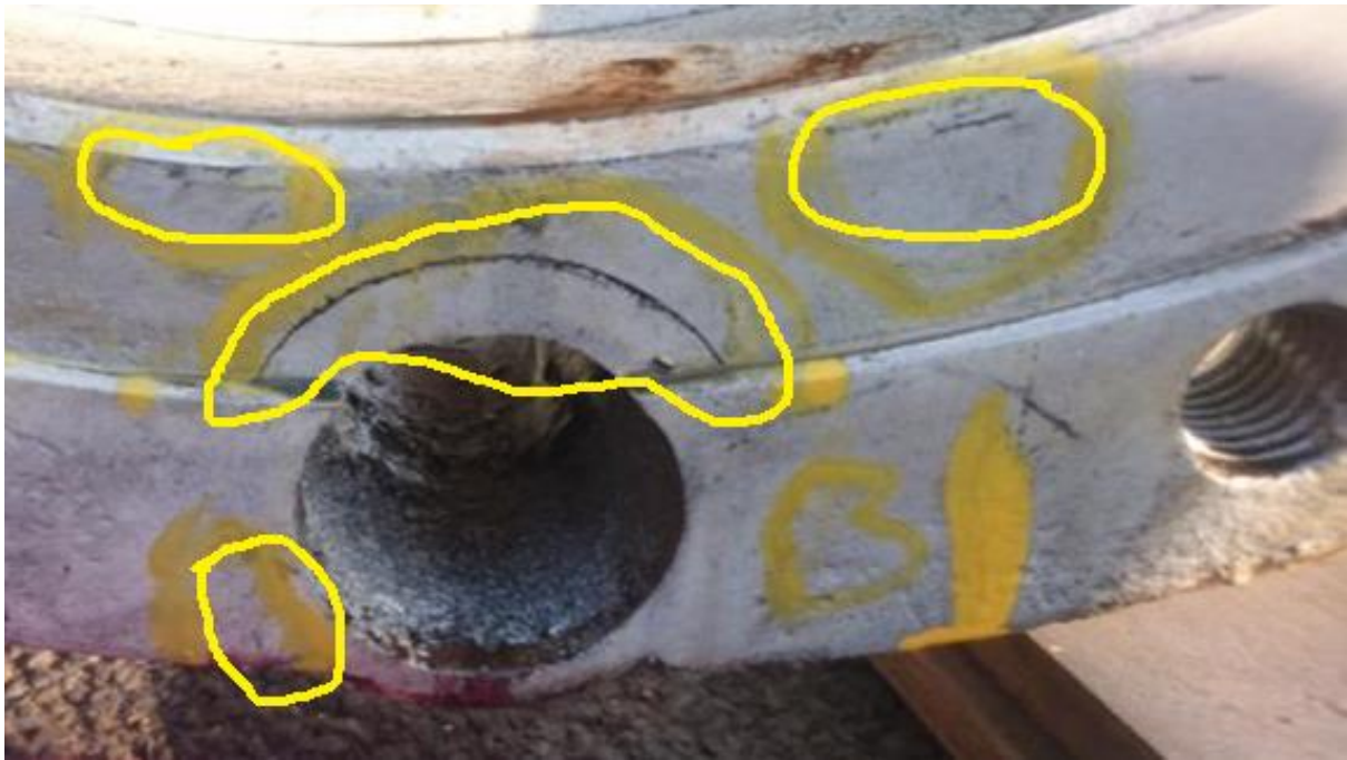
Axle A-Frame spring bolt boss cracking (mpi)
